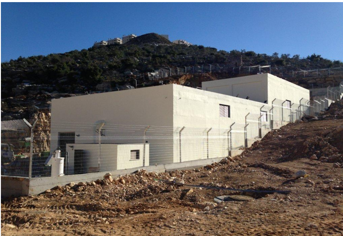
Photo 3.2: Alteera Wastewater treatment plant
